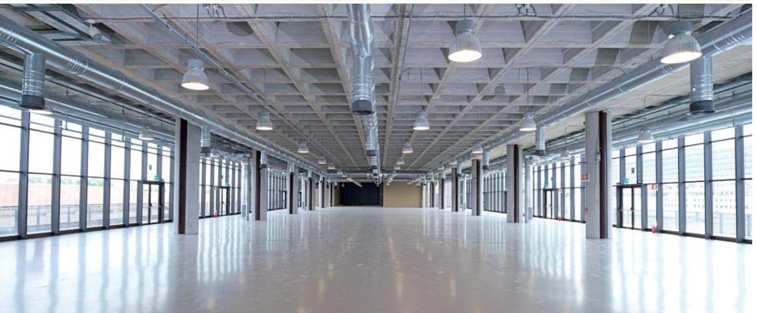
4F 1 curtain wall with Corten steel mullions and transoms, that integrates EBE thermal break door and window frames used for entrances and emergency exits. The use of properly treated Corten steel provides interesting colour variations, creating a highly natural effect that is crucial to ensure the smooth integration of the building in the fragile lagoon environment.
