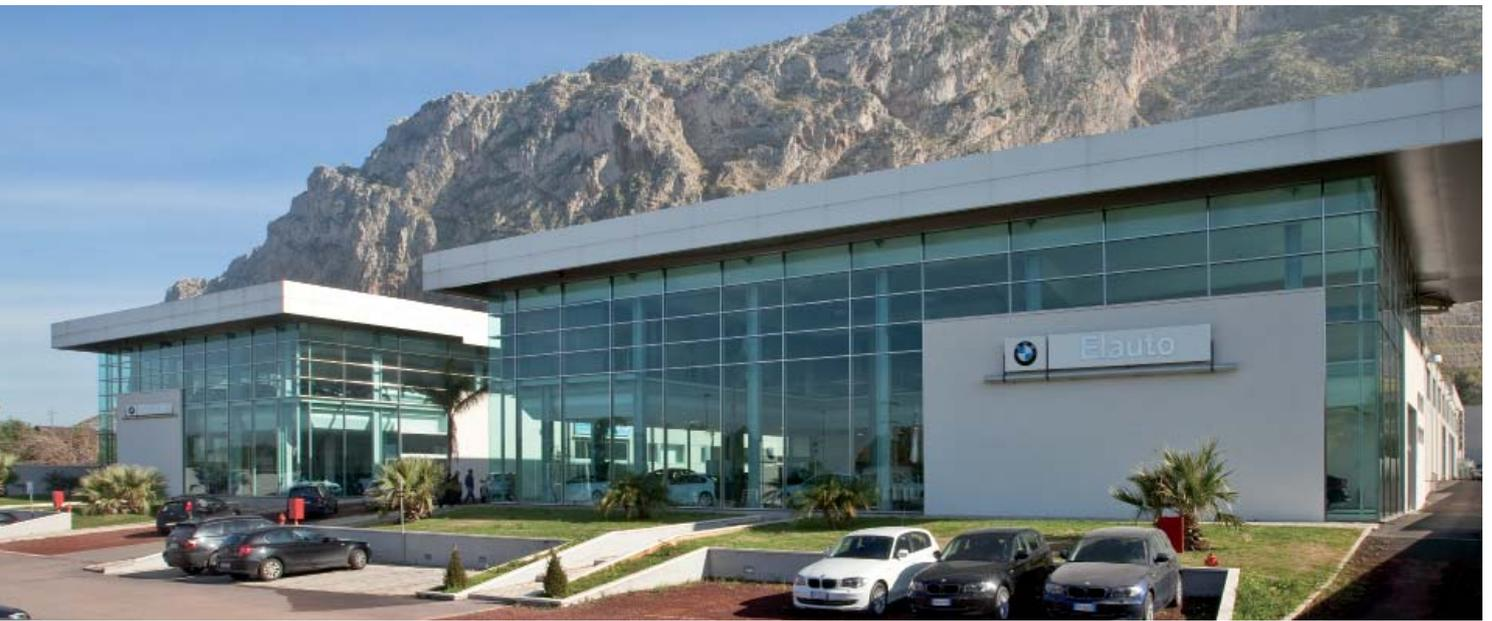
installed to support Secco Sistemi 4F 2 curtain wall with mullions and transoms in AISI 316L stainless steel. The modules of the glass window, in the first vertical order, have been cut to the maximum possible size for a glass plate. Sistemacciaio door and window frames made in AISI 316L stainless steel with a
